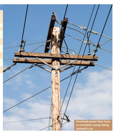
Step and touch potentials can occur when a tree trimmer or landscaper is working in an elevated position or on the ground near overhead lines. The location should be established such that the person and the longest conductive object he or she may contact cannot come within 10 feet for lines 50 kilovolts or less and more for higher voltages.
